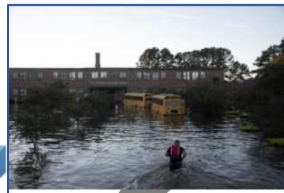
① Damage and loss; impacts of natural hazards on communities
