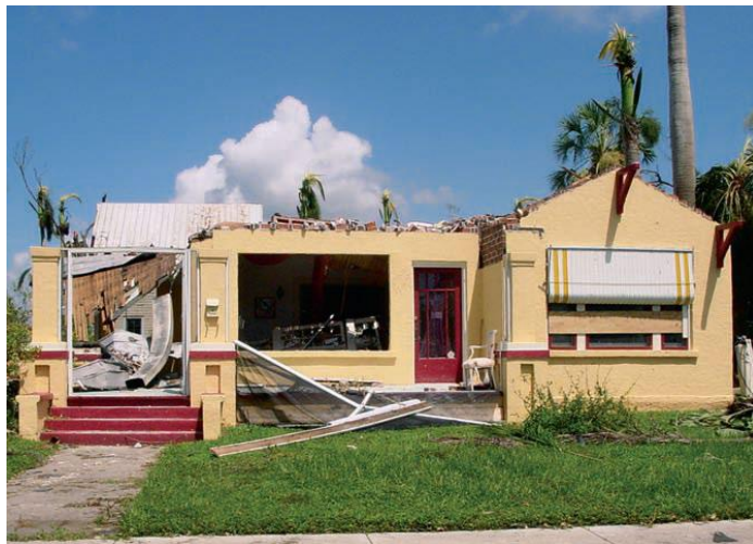
Roof failure from pressurization when the windward window failed. (FEMA 488)
